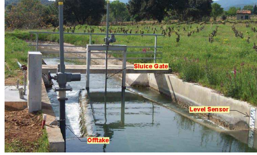
Figure 2: Upstream of the Avenq station with level sensor, offtake, and sluice gate with local controller.
